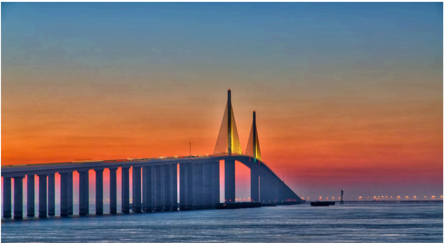
Tampa Sunshine Skyway Bridge
